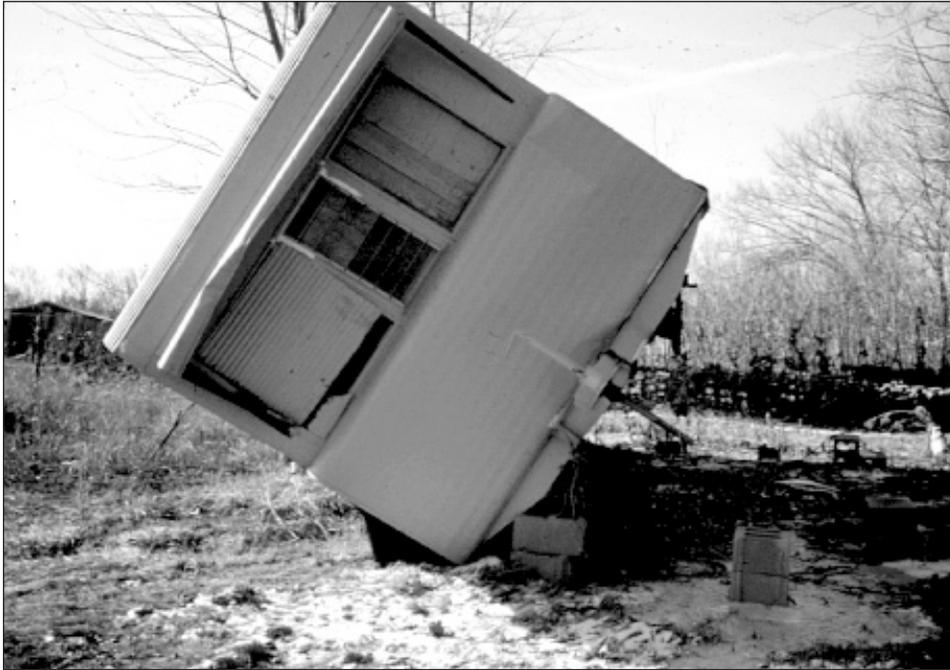
Figure 7-8. Failed foundation system that used masonry piers.
